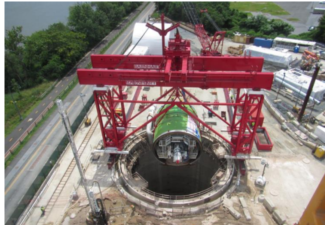
Tunnel Boring Machine, Nannie, Lowered into Shaft to Begin Mining
